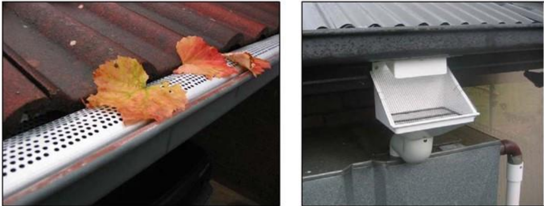
Figure 1.6: Gutters designed for pre-filtration of water from coarse bodies
