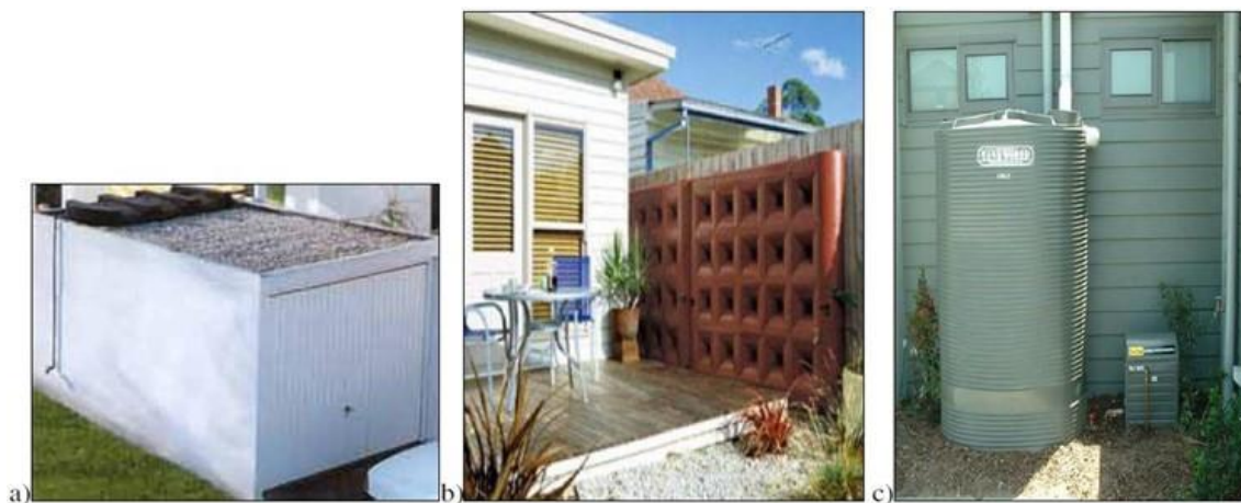
Figure 1.11: Examples of a) an above-ground 750-litre polyethylene tank, positioned on the cover of a box-garage; b) tank for minimum encumbrance; c) tank for irrigation use
