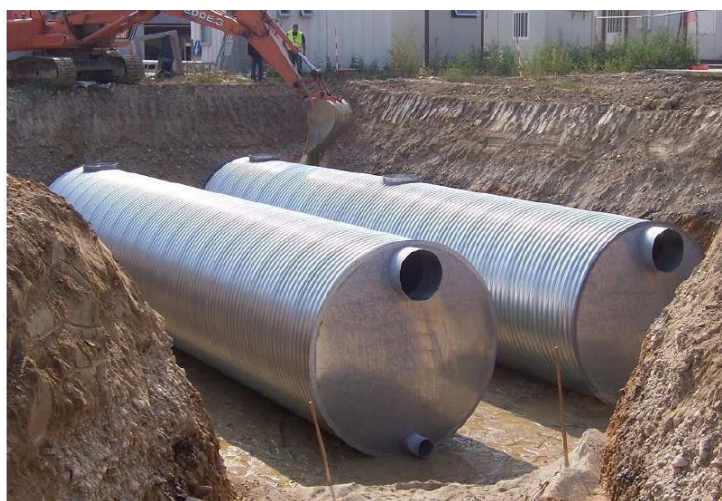
Figure 1.10: Steel tanks for water storage
