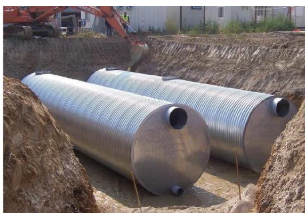
Figure 1.21: Steel tanks for storing rainwater
