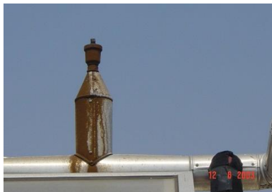
Figure 5.2: Inadequate air-vent and collector stagnation
