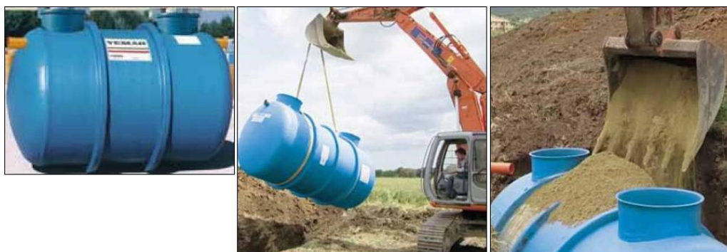
Figure 1.20: Fiberglass tank produced by Vemar and its installation
