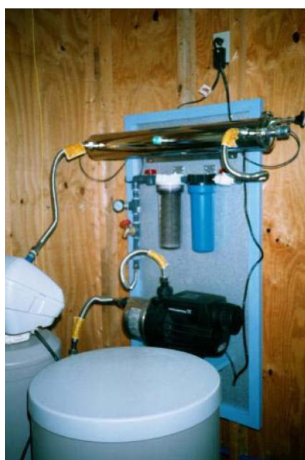
Figure 1.24: Typical treatment system with a 5 µm cartridge filter, a 3 µm active carbon filter and ultraviolet light debacterizer (left), and ultraviolet debacterizer (right)
