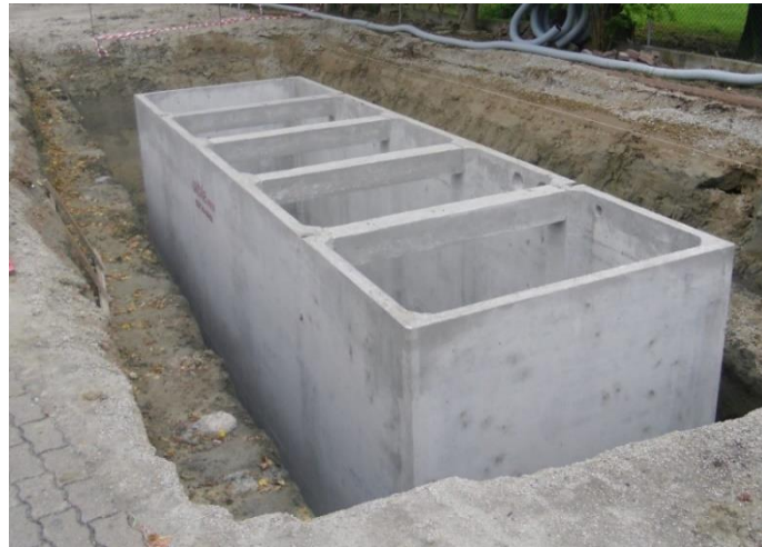
Figure 1.9: Concrete tank
