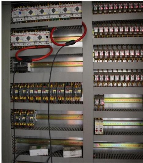
**Figure 1.7: Two current clamps installed in an electric board**
