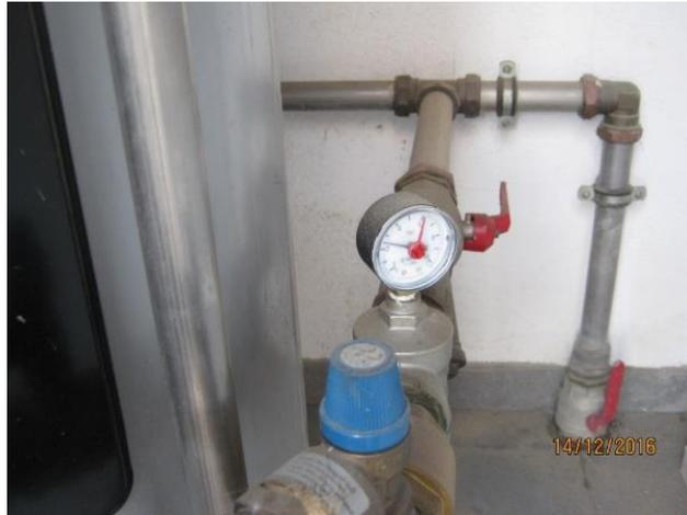
**Figure 1.5: Pressure gauge in a domestic hot water system**
