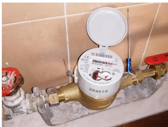
**Figure 1.1: Nutating disk flowmeter**
