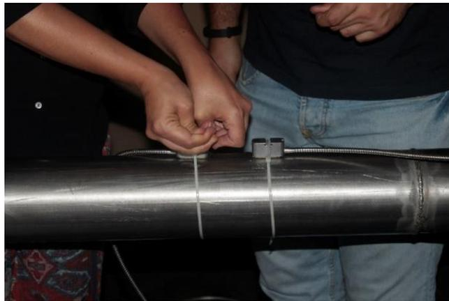
**Figure 1.3: Installation of ultrasonic flowmeter transducers/receivers**
